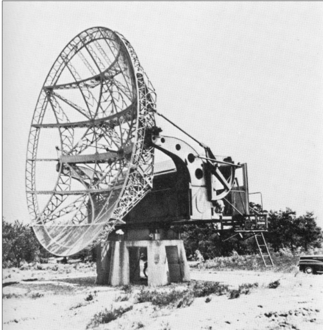
Figure 3: The Würzburg at Kootwijk used for observing the 21 cm HI line between 1951 and 1955.
