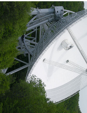
Effelsberg, Germany - 100m fully steerable telescope
