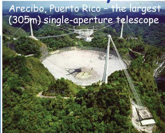
Arecibo, Puerto Rico - the largest (305m) single-aperture telescope
